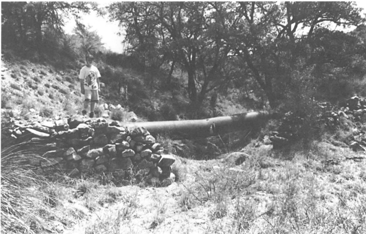
Kentucky Camp: typical 20" or 24" pipeline (support has been stripped away). Courtesy of the Coronado National Forest, Richard and Florence Lord, photographers.
