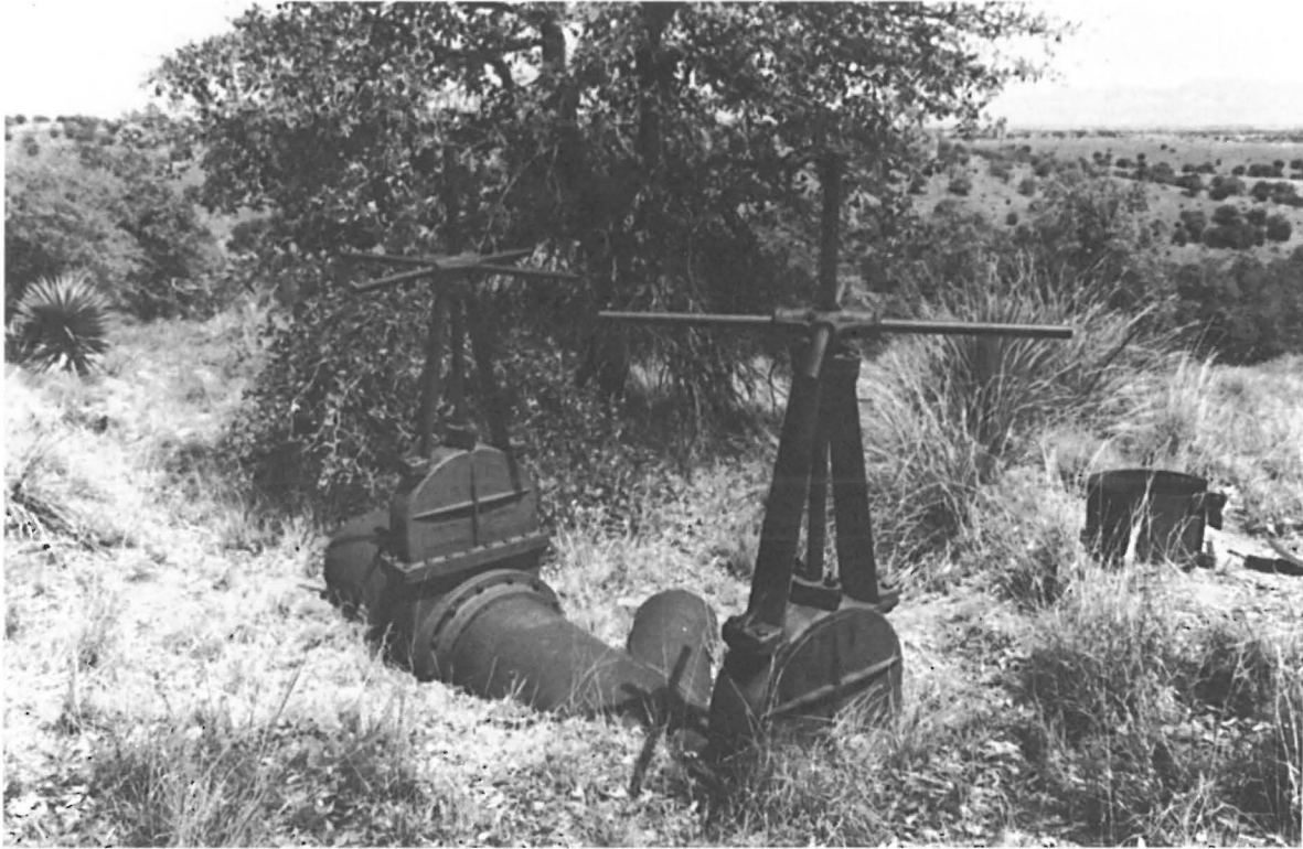
Kentucky Camp: dual gate valves at "Y." Courtesy of the Coronado National Forest, Richard and Florence Lord, photographers.
