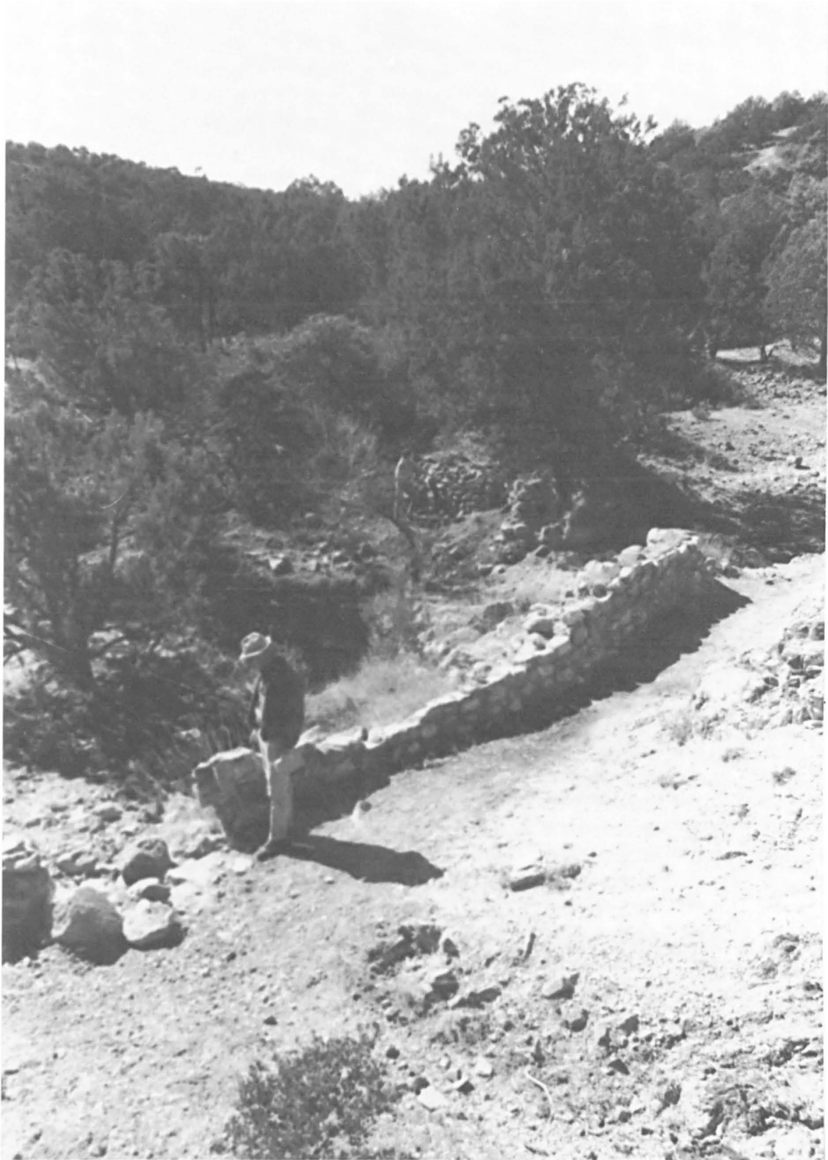
Kentucky Camp: remainder of Stetson's Dam. Man is standing in path of water from retention basin to continuing ditches, and examining what had been a waste gate. Courtesy of the Coronado National Forest, Richard and Florence Lord, photographers.
